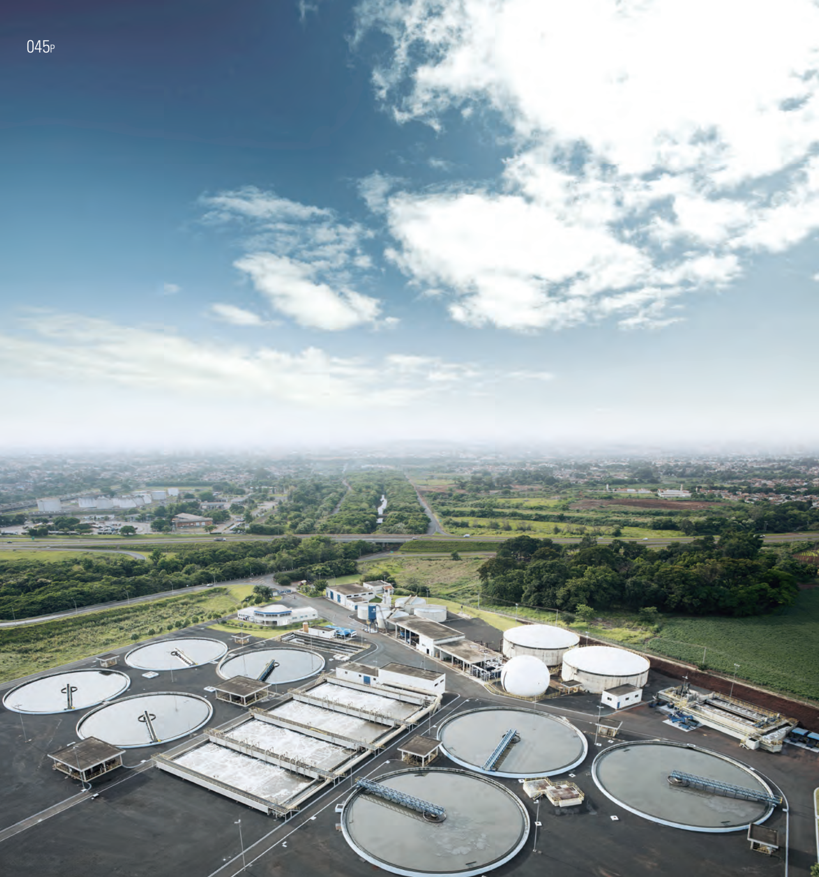
045P Ribeiro Preto Wastewater Treatment Plant Location : So Paulo, Brazil - 150,000 m³/d WWTP
