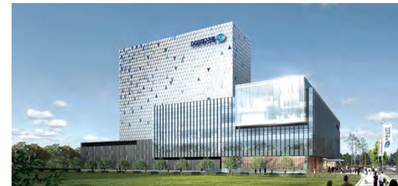
Daegu Bank (DGB) Data Center (PreCon)
