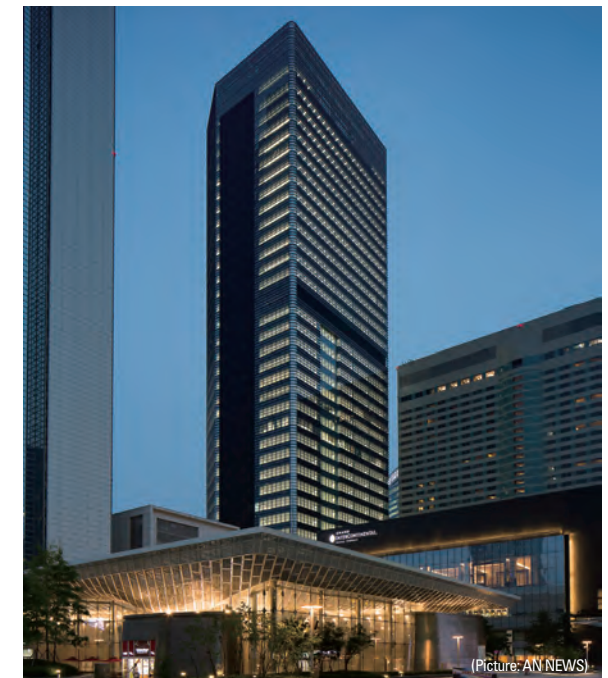
Parnas Tower (PreCon)
